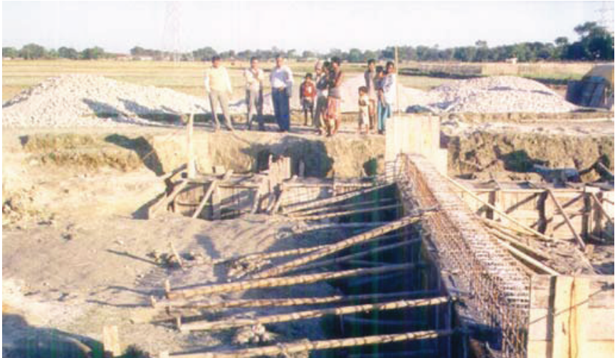
Figure 2. Constructing a gully plug to retain groundwater
