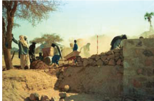
Figure 2: Construction of diversion works
