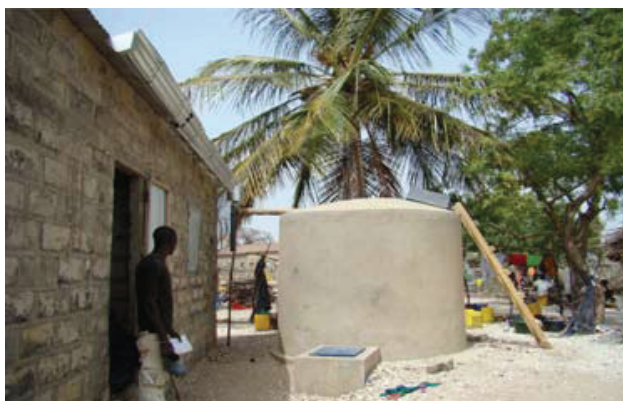
Figure 3. A rainwater harvesting tank being maintained in the village of Diogane
