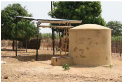
Figure 2. A hangar built by partner organization CCF as no appropriate roofs are available for roof water harvesting
