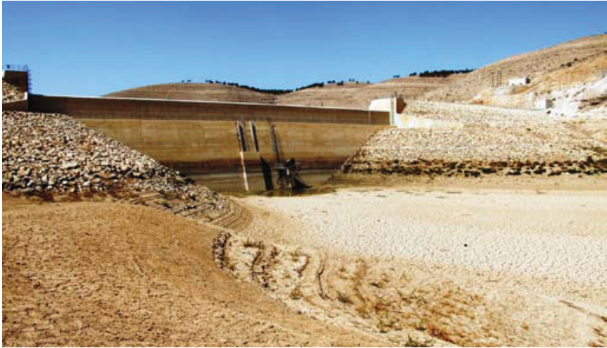
Figure 3: Sediment Accumulation at the Bottom of the Wadi Wala dam has lead to the Closure of the Bottom Outlet and the lower Draw-off Pipe
