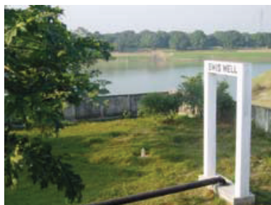
Figure 3. River bank infiltration well in Bangladesh for arsenic-safe water supply
