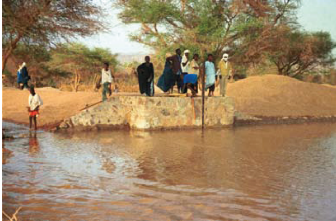
Figure 4: flood flow entering the infiltration basin
