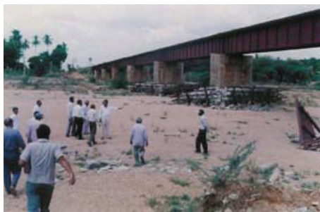
Figure 3. Railway bridge foundation frequently being repaired due to sand mining across Uttara Pinakini river in Gauribidanur taluk, Karnataka, 2002. (Hemalatha, A.C. et al. 2005)
