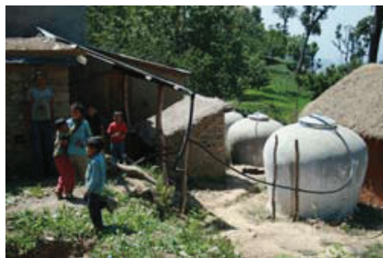
Figure 1. Rainwater harvesting tanks in Bubeyrakhe, Nepal
